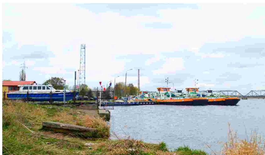
Icebreaker base, Karpia St. in Szczecin – present condition, a view from plot No. 7/16
